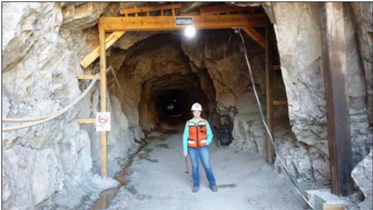
Photo 6-4: Main Portal at Babicanora, 4 m by 4 m, built in 1860's
