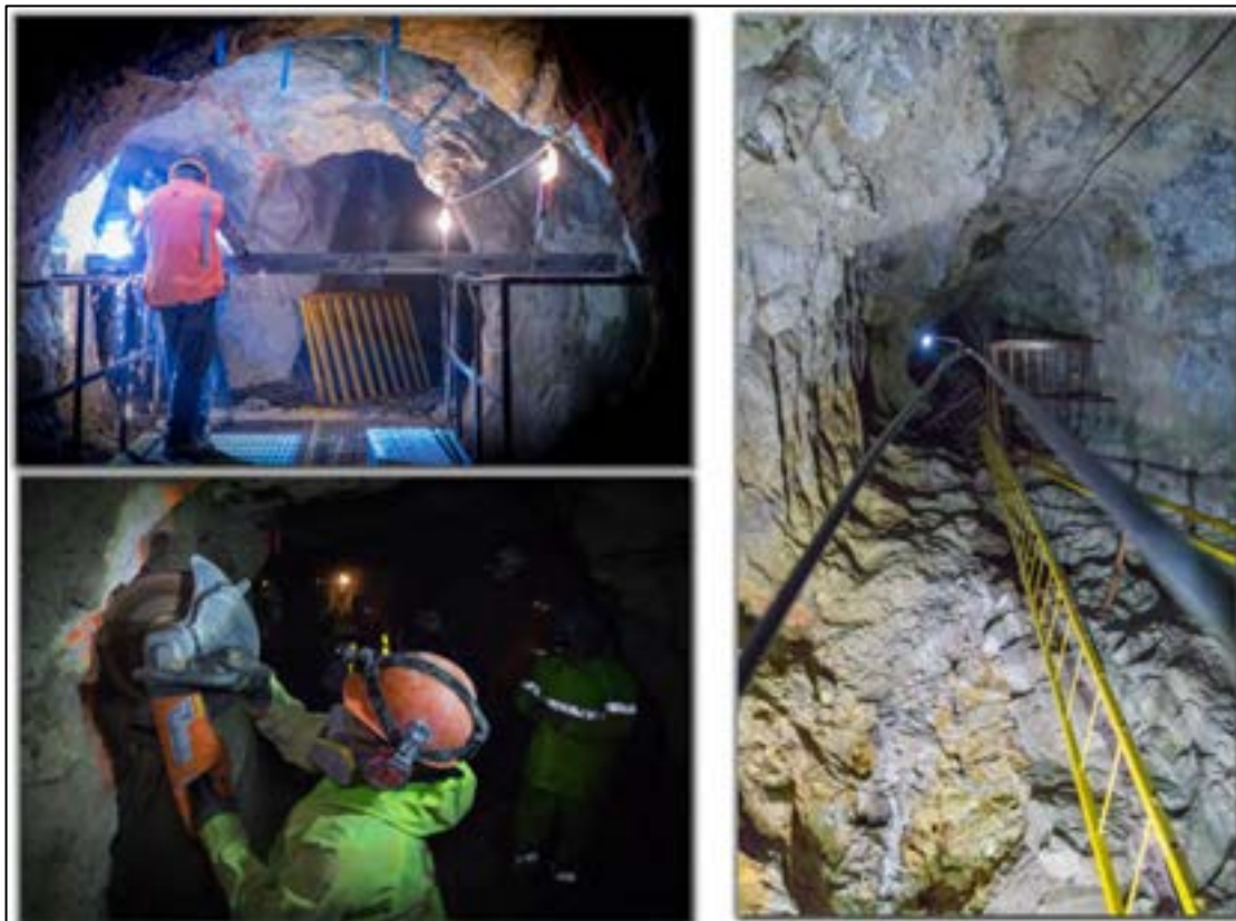
Photo 8-1: Photos of Las Chispas Underground Rehabilitation Activities
