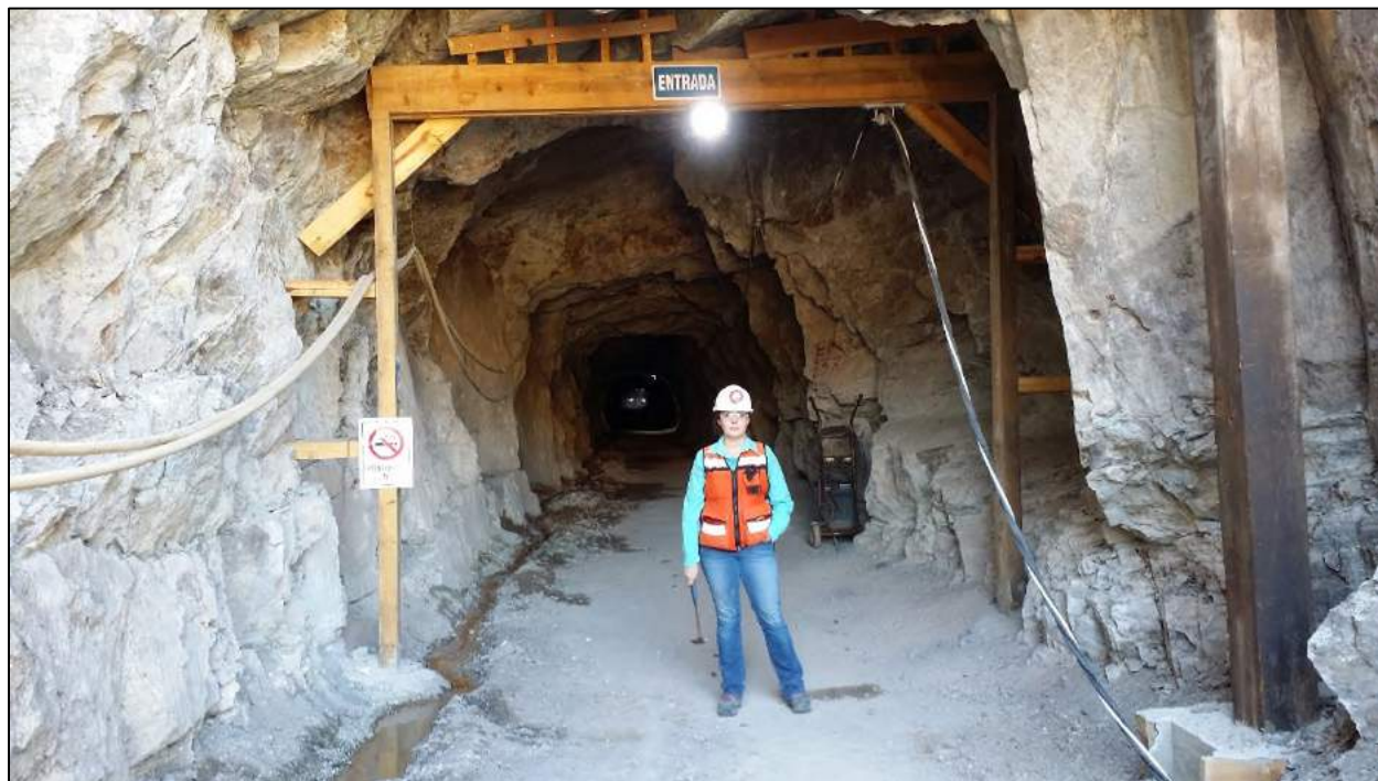
Photo 6-4: Main Portal at Babicanora, 4 m by 4 m, built in 1860's
