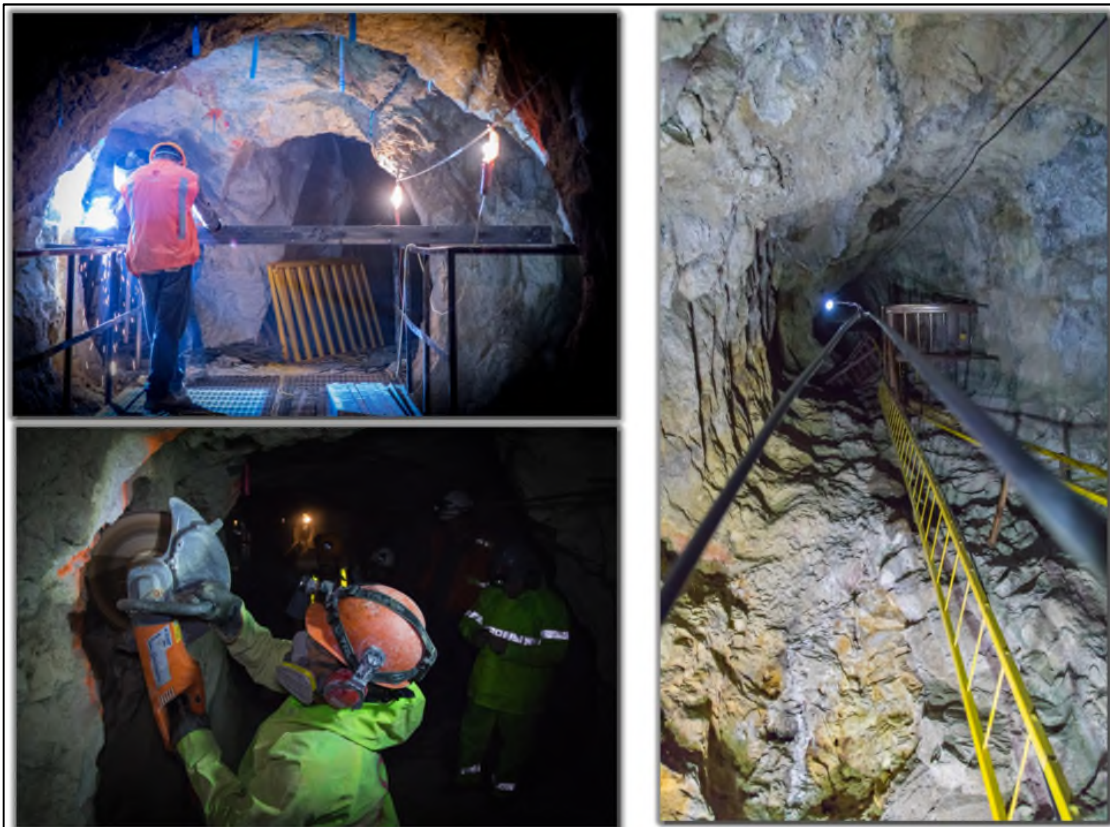
Figure 8-1: Photos of Las Chispas Underground Rehabilitation Activities
