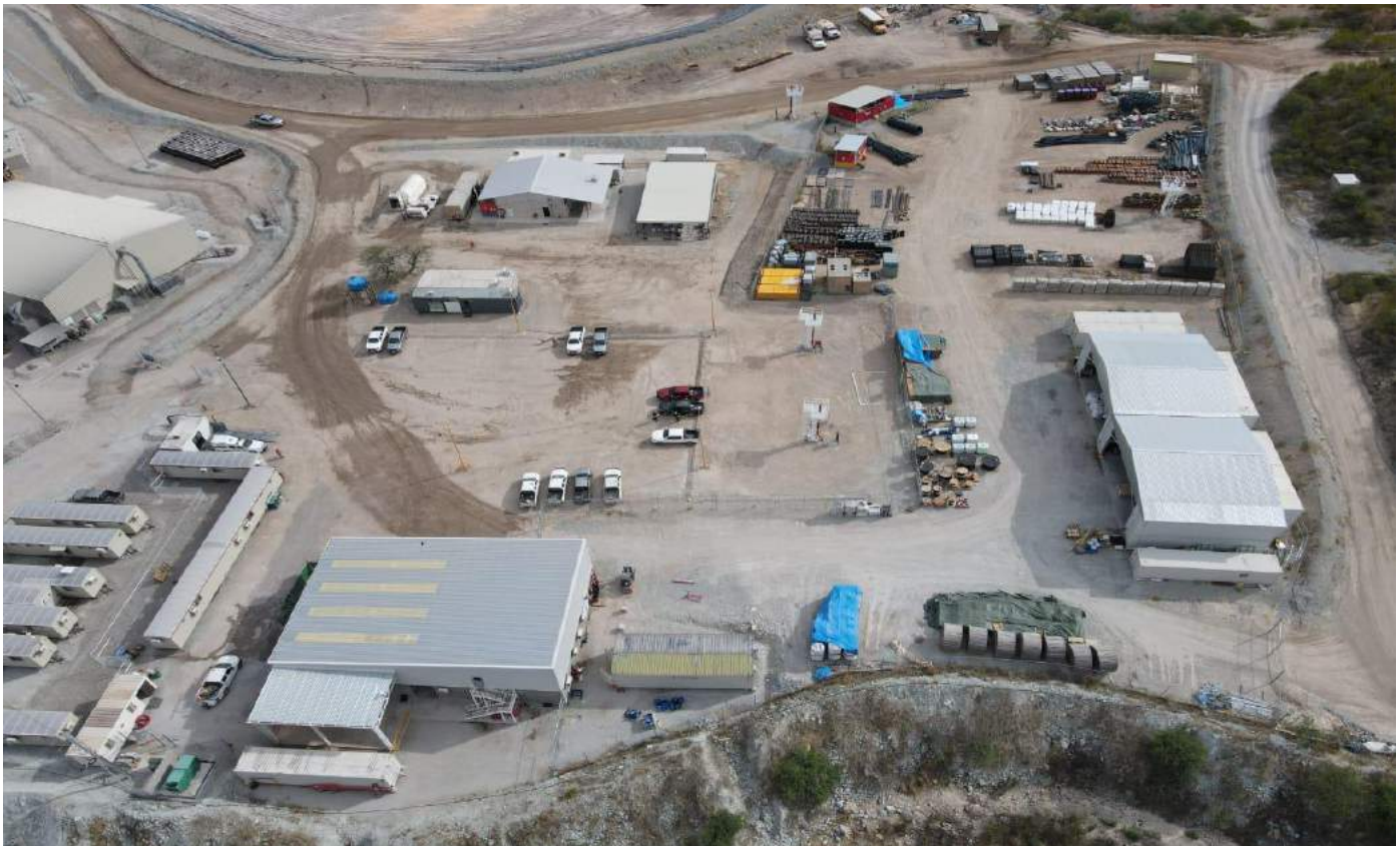
Figure 18-23: Warehousing Facilities with the Main Warehouse (lower left corner)
