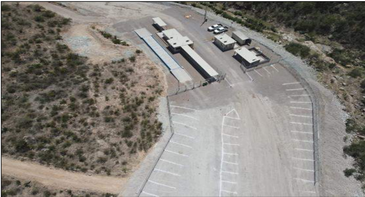
Figure 18-5: Security Gate #2 (Main access point)
