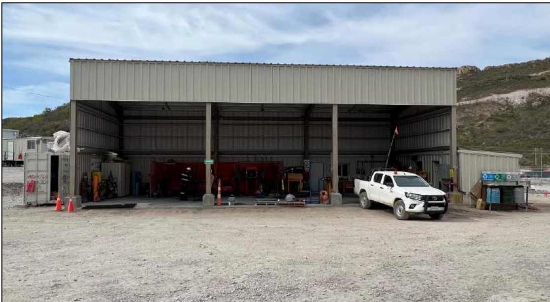
Figure 18-26: Process Plant Maintenance Shop
