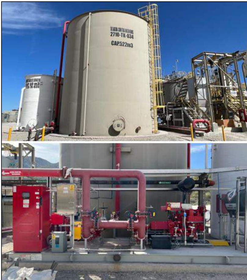
Figure 18-14: Fire Water Supply and Distribution Systems
