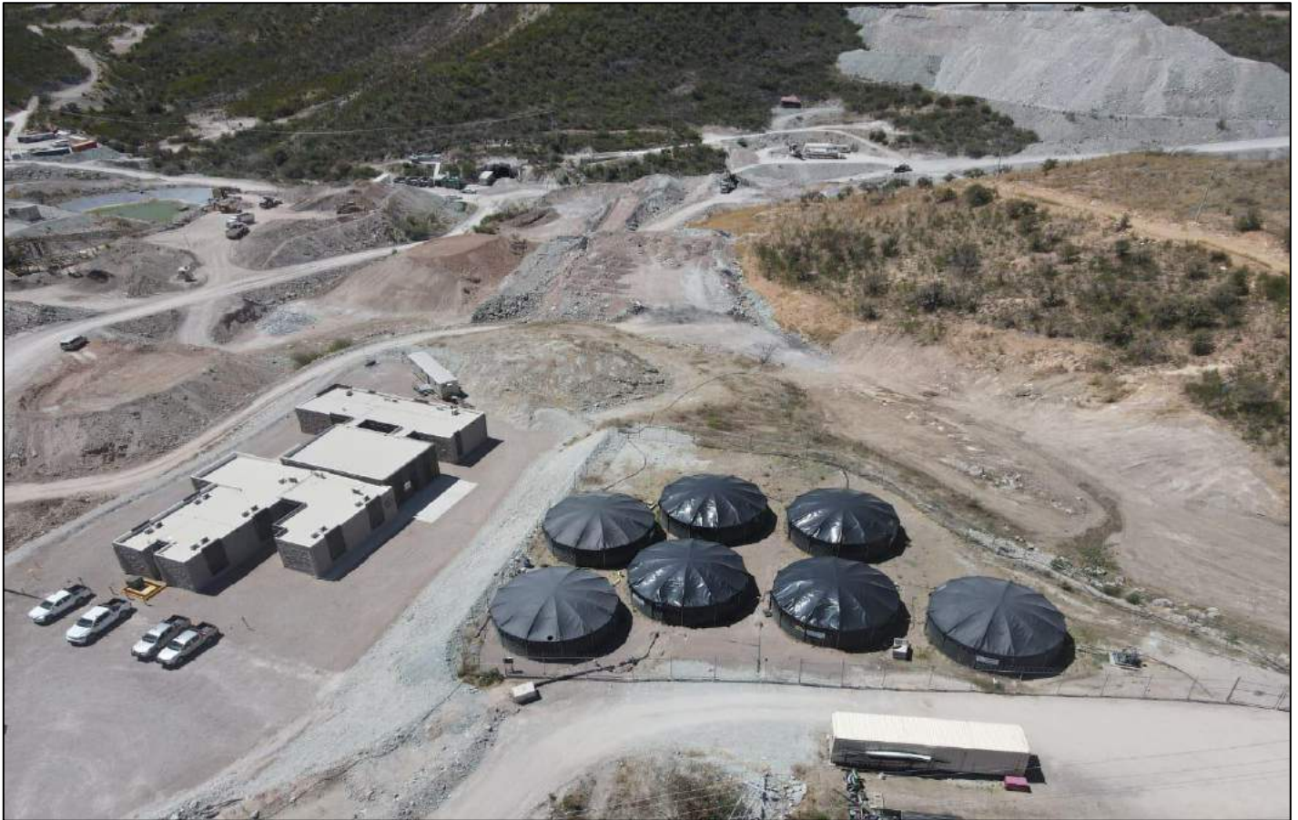
Figure 5-2: Water Distribution Tank Located Near the Main Office
