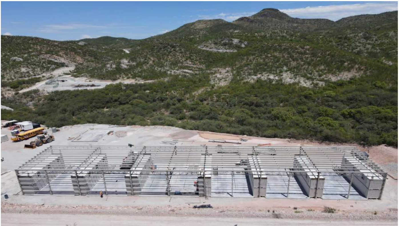
Figure 16-32: Surface Maintenance Shop – Construction View
