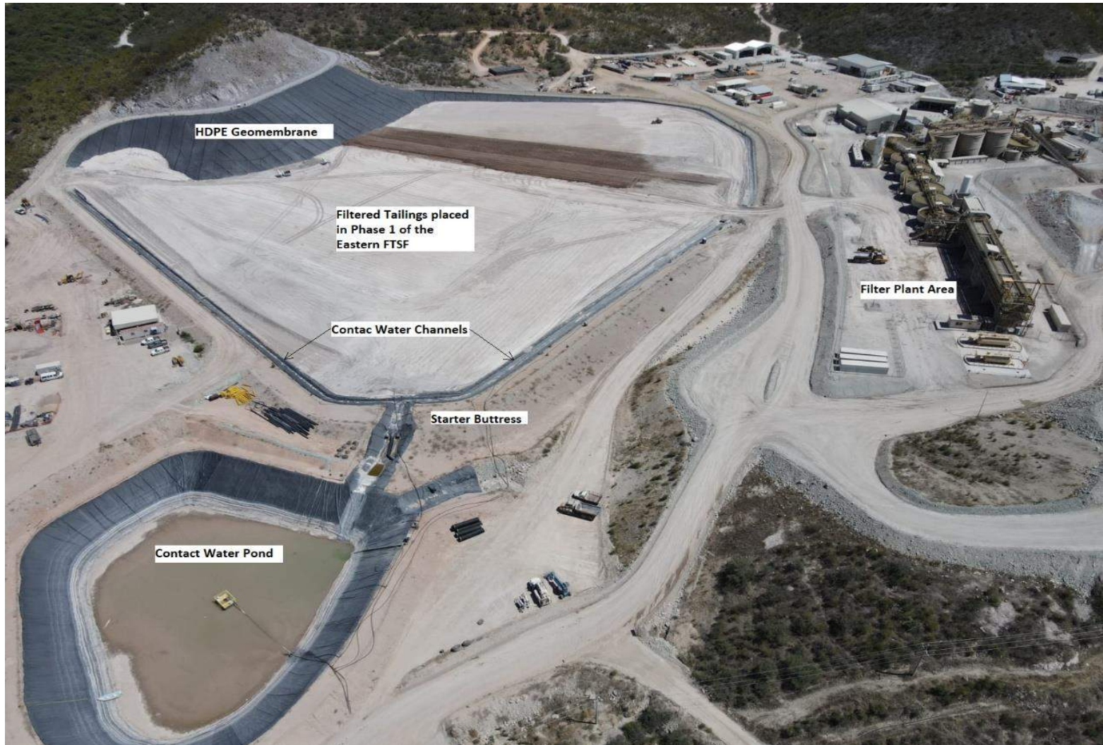
Figure 18-34: Aerial view of the existing East FTSF - Phase 1 and associated Contact Water Pond
