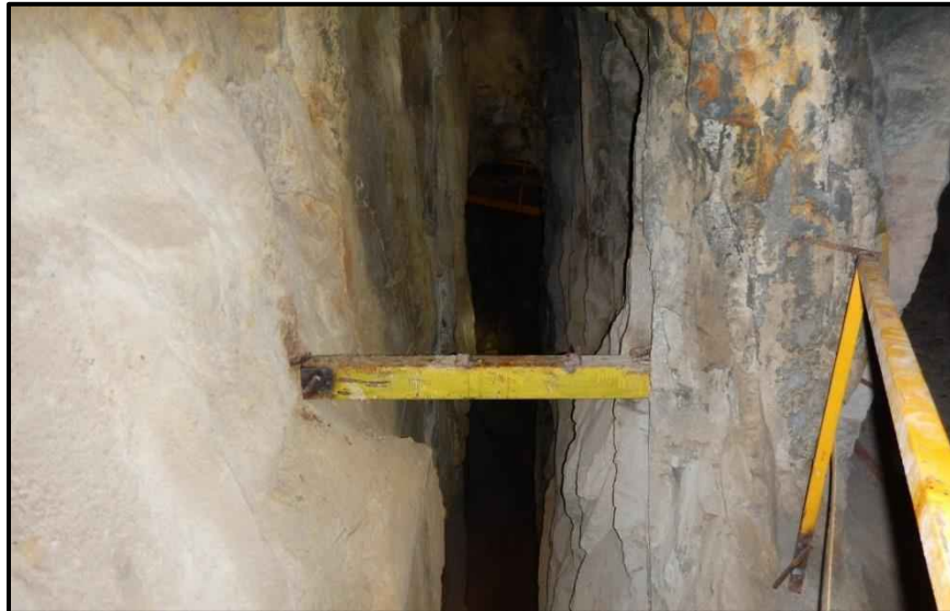
Photo 16-1: Historic Mined-out Area Showing Stable Ground Conditions
